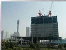
New HQ building under construction(April, 2008)
